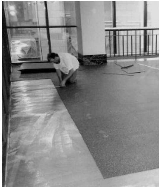
Square Cut Glue Down Installation
